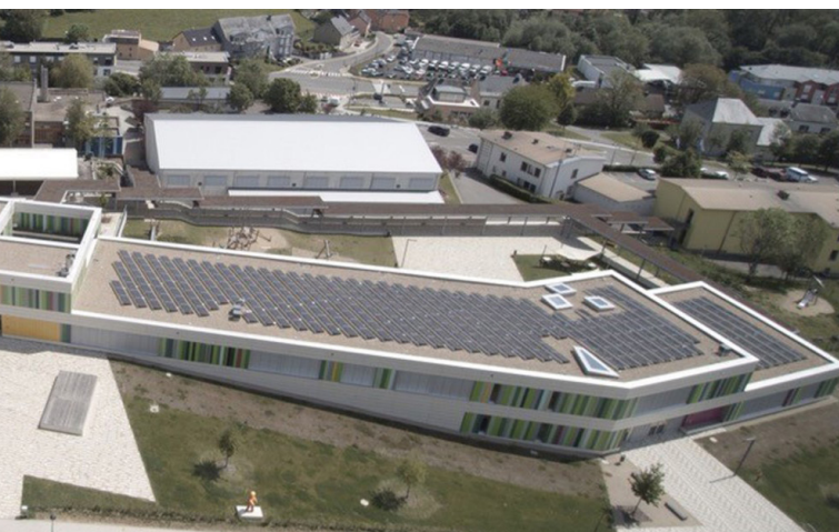
Photos : Campus scolaire Schouweiler © WW + Architektur & Management SARL
